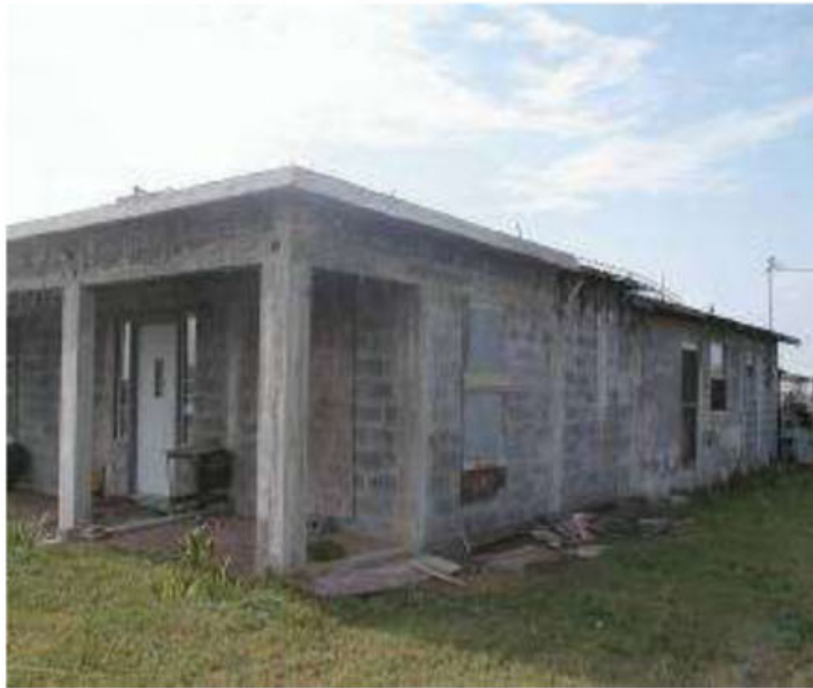
House almost finished
