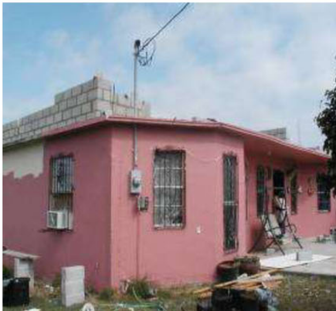
Building second floor
