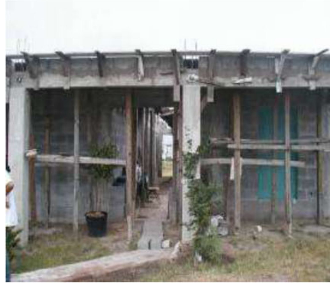
House under construction
